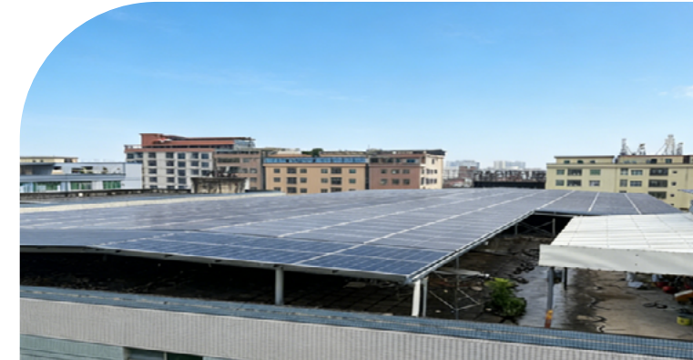
Solar panels at our manufacturing plant in China.
